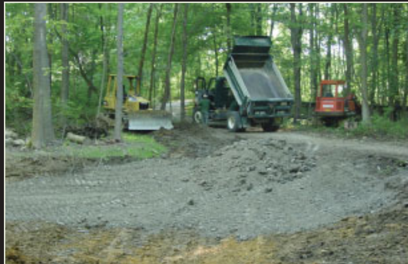
Lake Metroparks' newest vernal pool was created at Penitentiary Glen Reservation in fall 2005. A clay liner was added to prolong the pool into summer.
